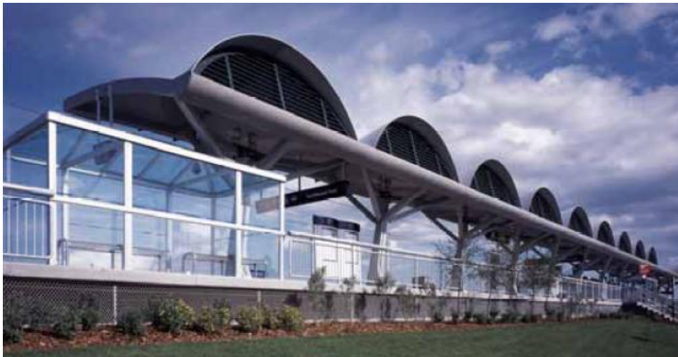
Figure 2.34. Shawnessy LRT station with UHPC canopies (Perry 2006)
