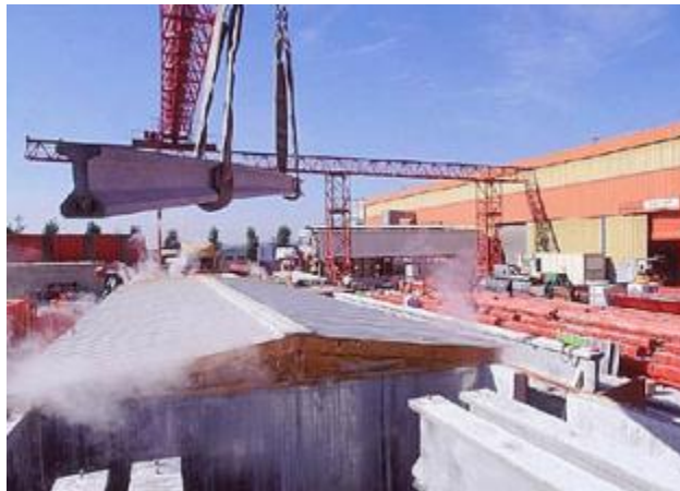
Figure 2.31. View of precasting area for UHPC beams for Cottenom Nuclear Power Plant (Lafarge North America 2007)
