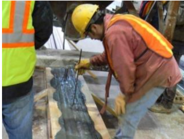
Figure 4.24. “Rodding” through the web of UHPC to eliminate formation of possible air pockets
