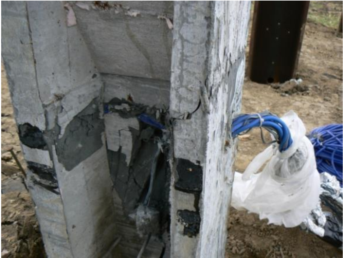
Figure 5.48. Bundle of instrumentation wires passing through the web and out of the flange of UHPC pile P1
