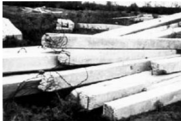
Figure 1.2. Precast, prestressed concrete piles damaged during hard driving (DiMillio 1998)
