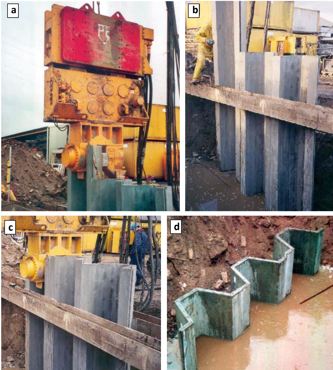
Figure 2.44. Views of a) to c) the driving process for SCFRC sheet piles and d) the completed view (Walraven 2007, Walraven and Schumacher 2005)
