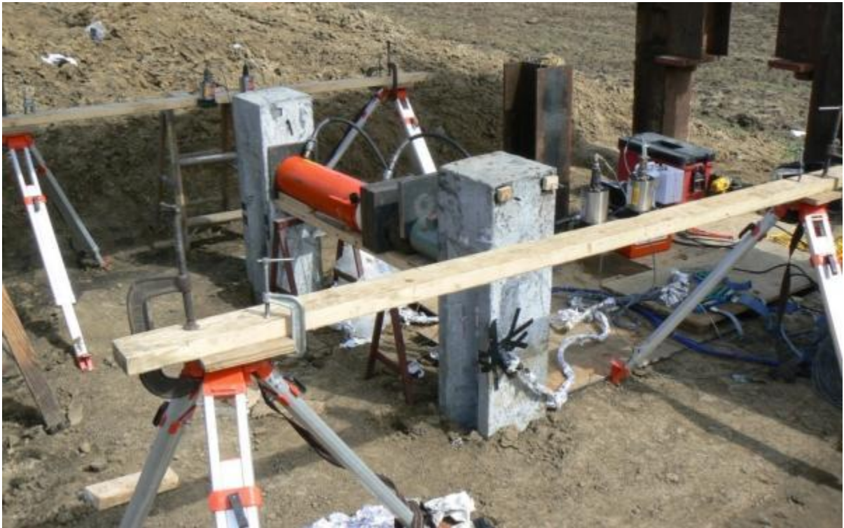
Figure 5.33. Overall layout at beginning of lateral load test on UHPC piles
