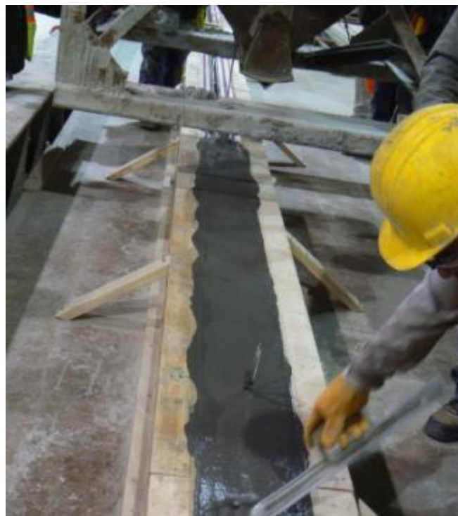
Figure 4.19. Pouring of 35-ft (10.7-m) long UHPC pile P1
