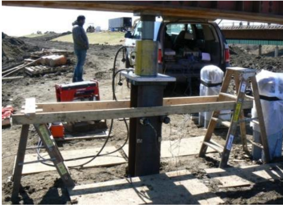
Figure 5.19. Wooden reference beams supported by ladders (steel pile)
