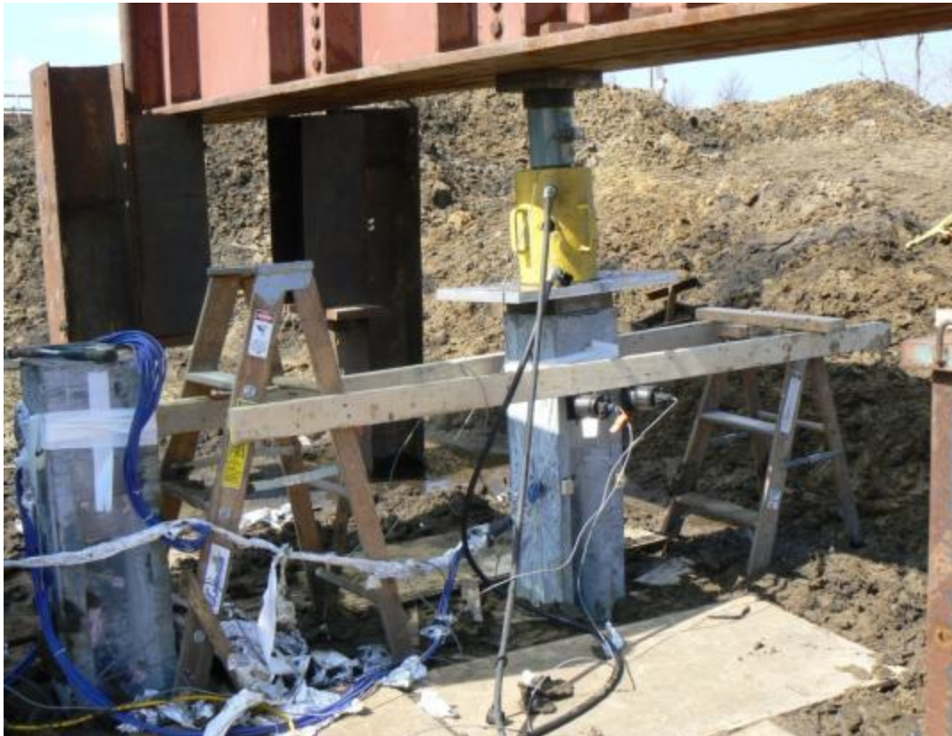
Figure 5.21. A view of the UHPC pile P1 during vertical load test 1
