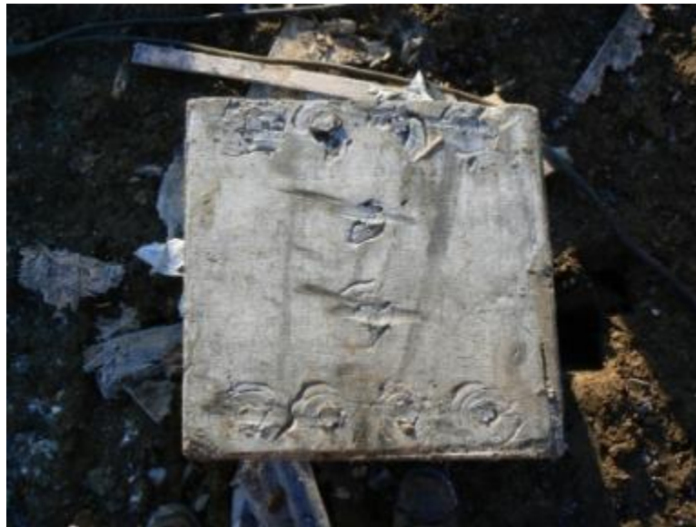
Figure 5.13. Condition of pile head at the end of driving pile P1
