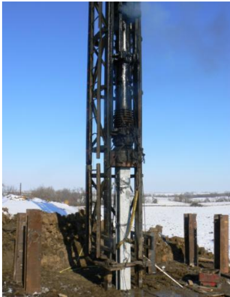
Figure 5.10. First UHPC pile being driven at the Oskaloosa test site
